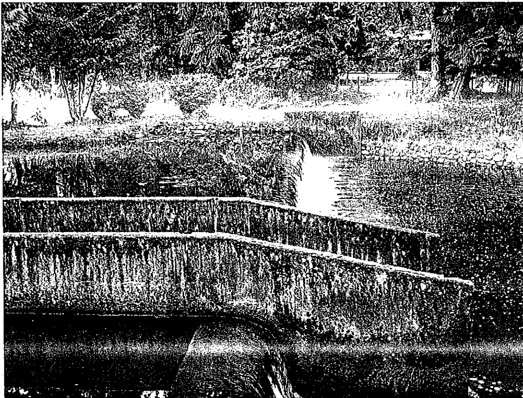
Fish Passage and Crest from Right Abutment
