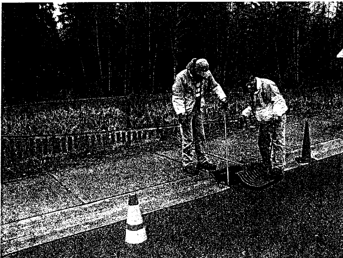
City workers inspect a catch basin that discharges into a storm pond
