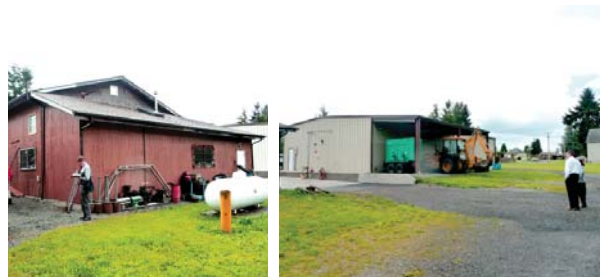
Public Works shops and equipment storage
